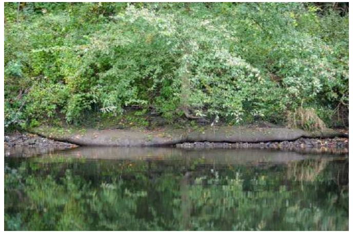
2024 CRC Site 8 (25) Notching forming above protected toe – this demonstrates the concern about holding the impoundment at higher average elevations than in the past.
