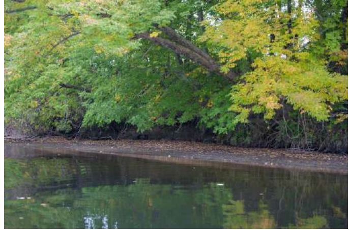
2024 CRC Site 9 (17) Exposed roots at bank toe
