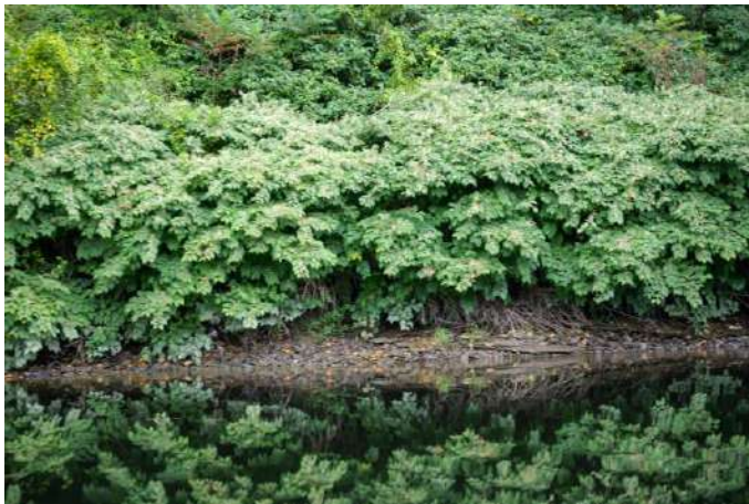
2024 CRC Site 8 (31) – knotweed overtaking repaired section
